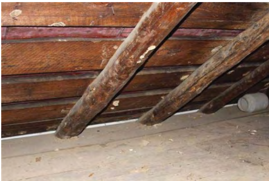
Rafter Connection At Attic Floor
